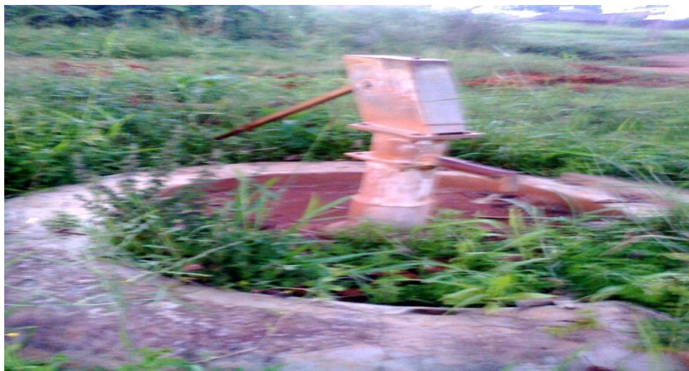
Figure 2: Non -functional shallow well in Obwola village
