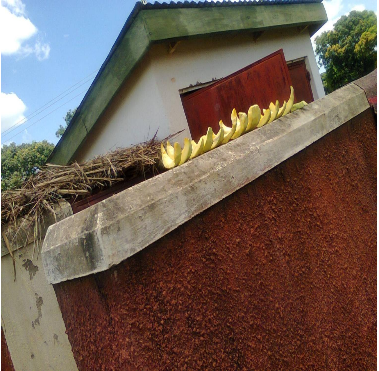
Pictoral: One of VIP household latrines belonging to the landlord in Puranga Trading centre. B in Parwech Parish. It has permanent walls, metallic well fixed doors and a corrugated iron sheets roof
