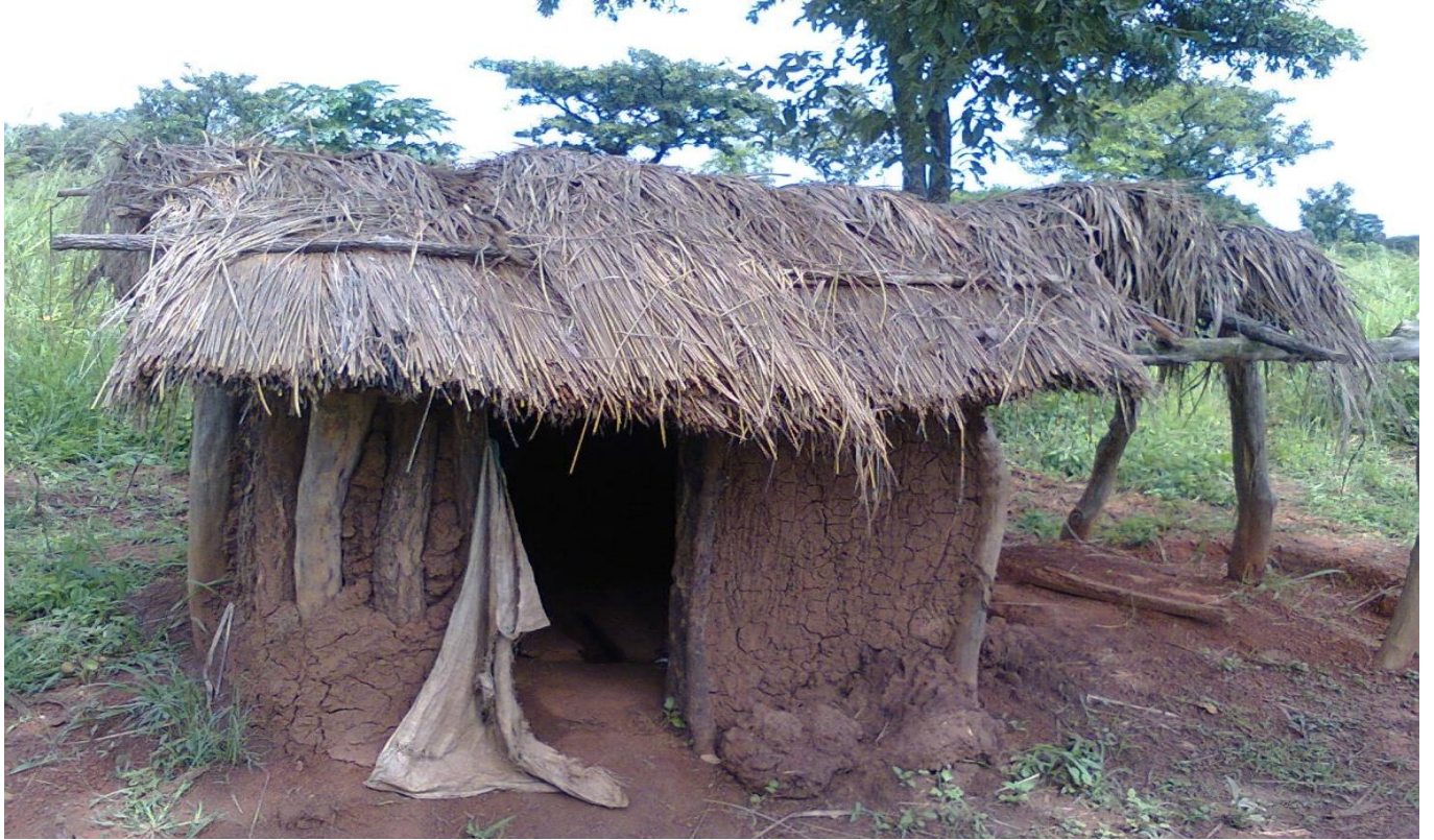
Pictoral: One of the household latrine of poor quality observed in Loborom Village in Oret Parish. It as a leaking roof, weak walls, no fitting doors and a busy surrounding compounds
